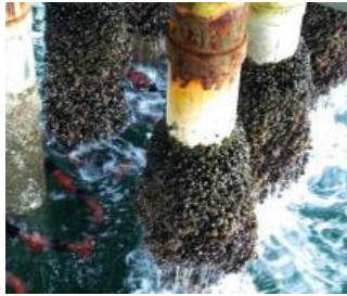
Figure 1 - Accumulation of marine growth
